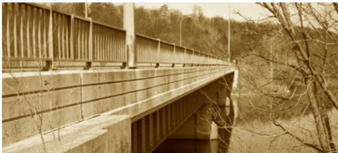
Mill Avenue Bridge
