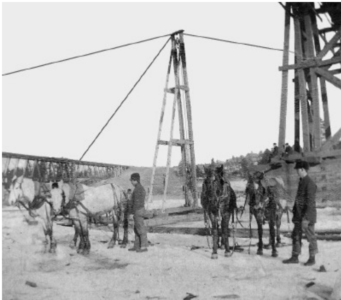
Building the Laurel Street Wagon Bridge, ca. 1883. Courtesy of Crow Wing County Historical Society
