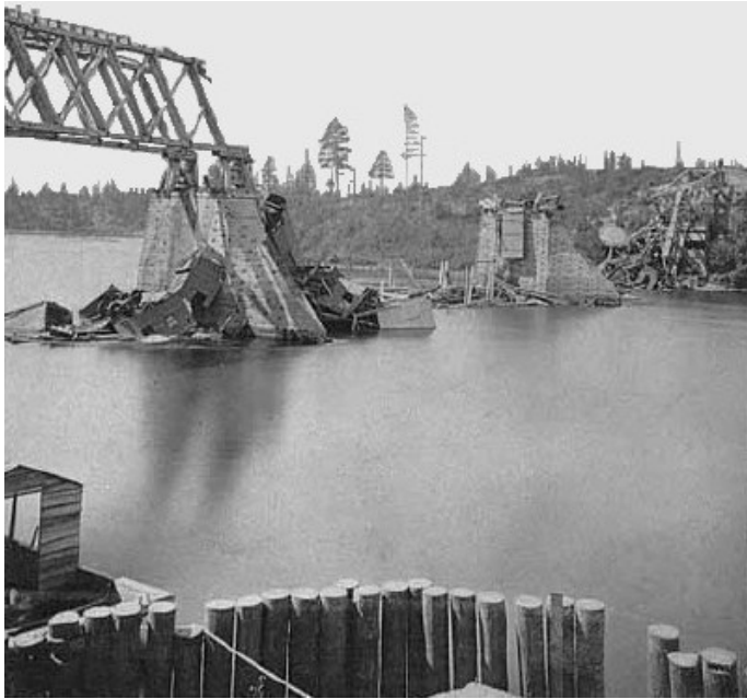
Northern Pacific Bridge Collapse, July 27th, 1875. Courtesy of Minnesota Historical Society
