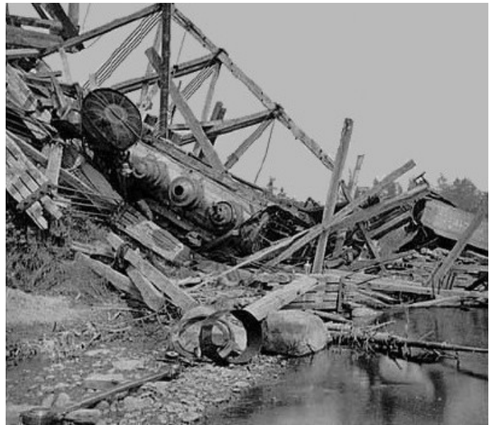
Northern Pacific locomotive lying on the west bank of the river after the bridge collapse, July 27, 1875. Courtesy of Minnesota Historical Society
