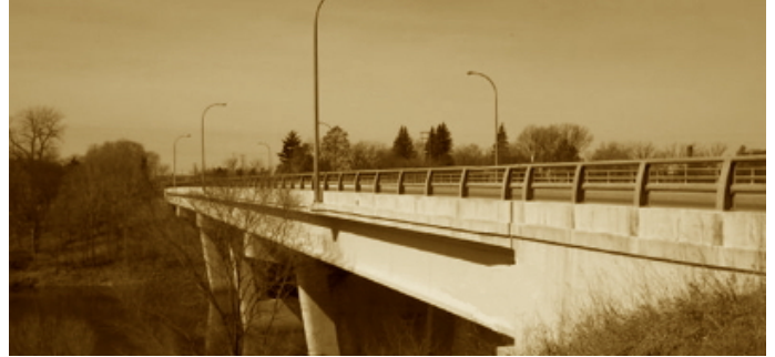
Laurel Street Bridge
