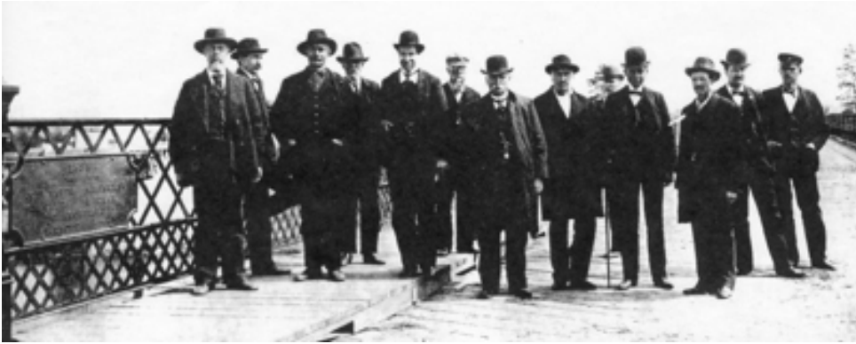
Laurel Street Bridge dedication, 1898. Courtesy of Crow Wing County Historical Society
