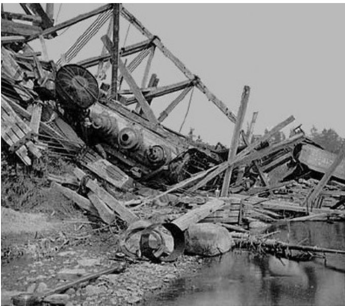
Northern Pacific locomotive lying on the west bank of the river after the bridge collapse, July 27, 1875. Courtesy of Minnesota Historical Society
