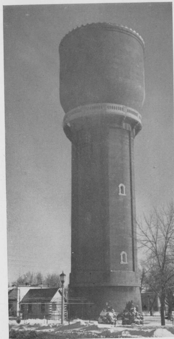
Photo by Ward Trask, Brainerd Brainerd's concrete elevated water tank. A distinguishing landmark for many miles around.
