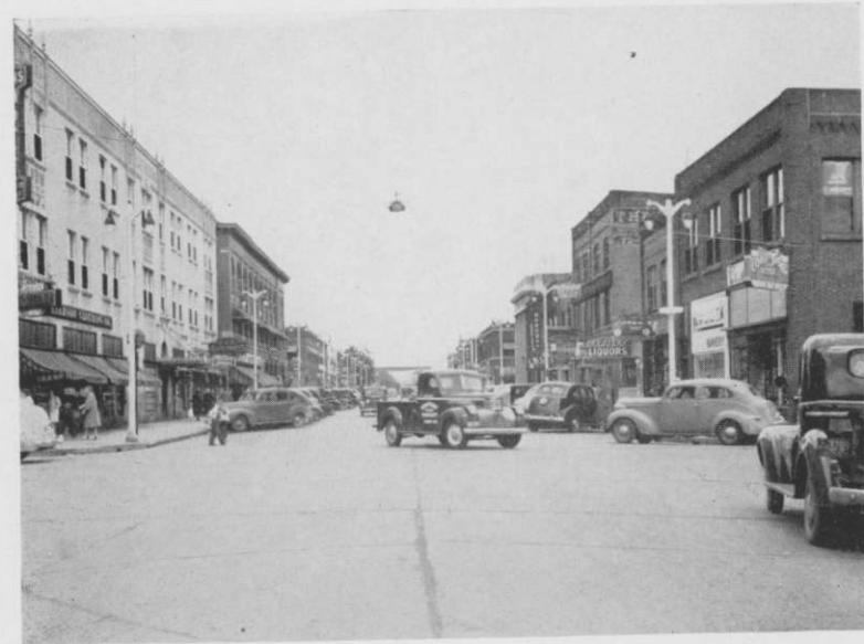
Photo by Ward Trask, Brainerd Laurel Street, looking east from corner of South Sixth and Laurel.
