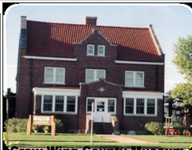
Crow Wing County Museum & Research Library Restored Sheriff's Residence
