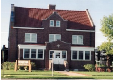
Crow Wing County Museum & Research Library Restored Sheriff's Residence
