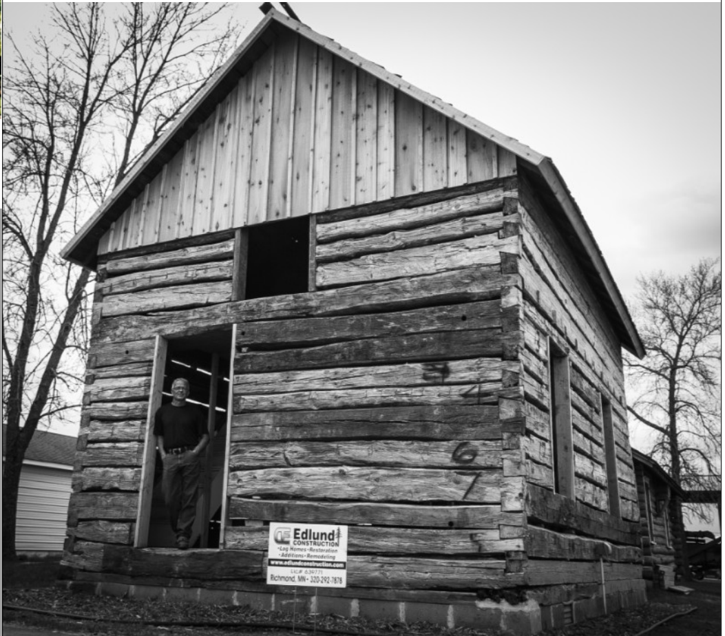
Pictured is Dale Edlund with Edlund Construction in the Carbine House
