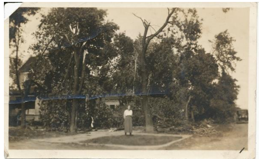
After a tornado near Gregory Park, 1919.
