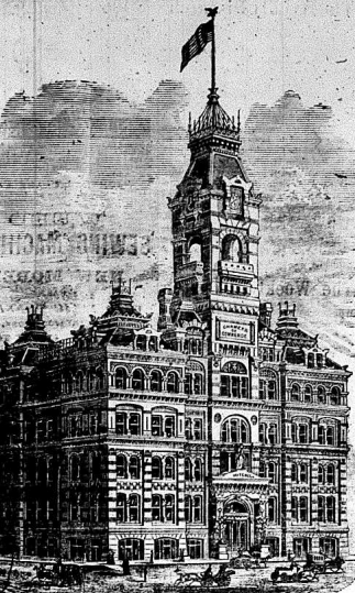
NEW CHAMBER AT CORNER OF MILWAUKEE
